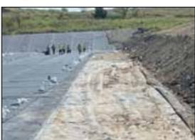
Workers completed the installation of a flexible membrane liner at the Coffey County Landfill. The \$200,000 liner was placed on the floor and walls of the newly constructed Cell No. 4, which is a 3.9-acre lateral expansion of the landfill. The new cell, scheduled to go into service early in 2021, will have an estimated lifespan of six to seven years.
